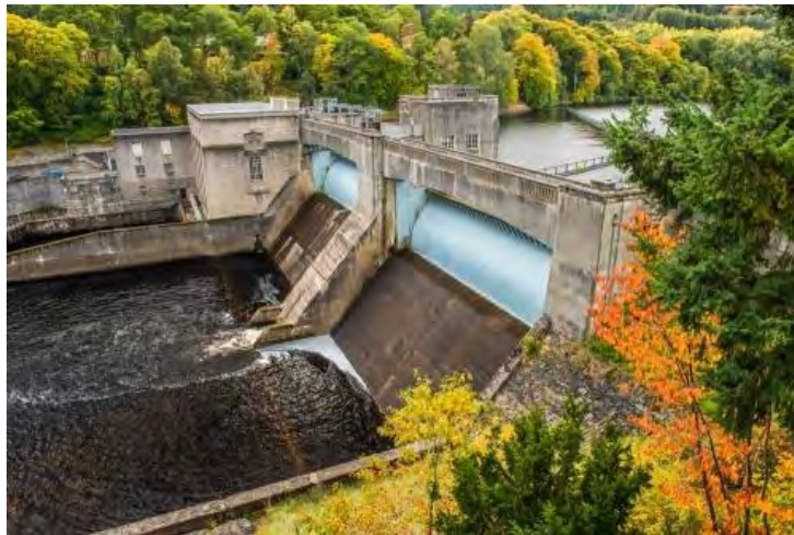
Figure 10: Pitlochry Hydropower Plant
