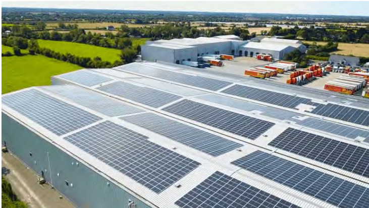
Figure 17: Commercial Solar Panel Installation. Source: Enerpower
