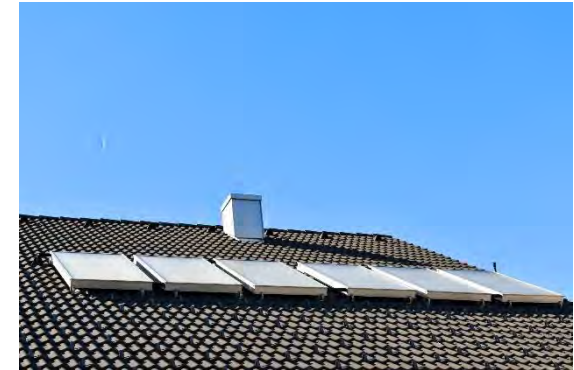
Figure 22: Flat plate collectors - fixed on the roof tiles or integrated into the roof
