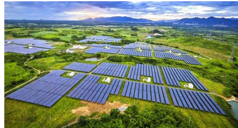
Figure 16: A Solar Farm. Source: The EcoExperts
