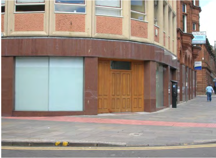
Inactive façade, John Finnie Street
