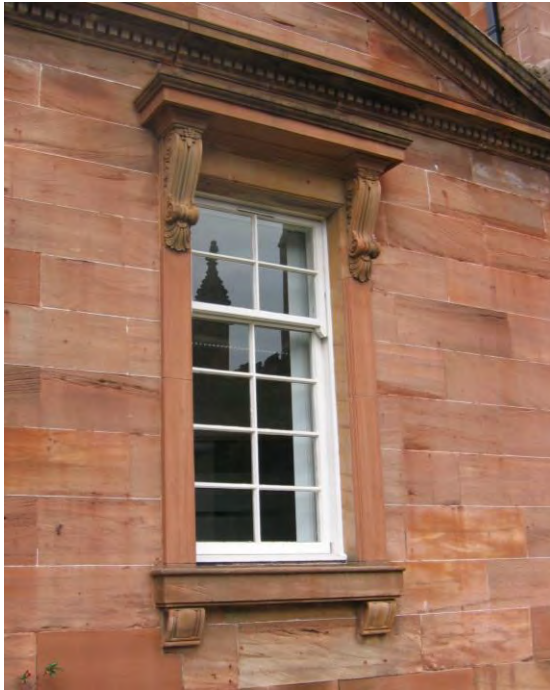
Sash and case window
