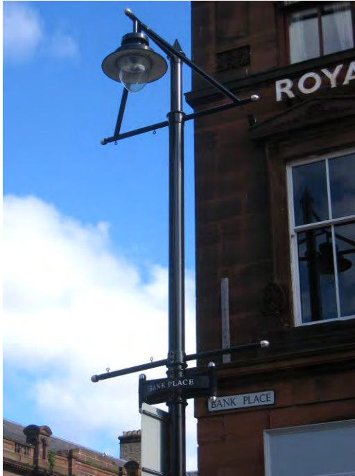
Street Lighting, Bank Place
