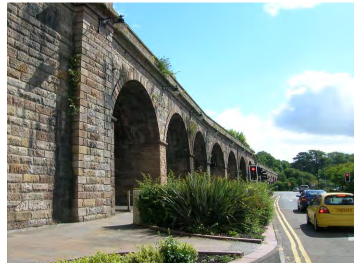
Kilmarnock Railway Viaduct
