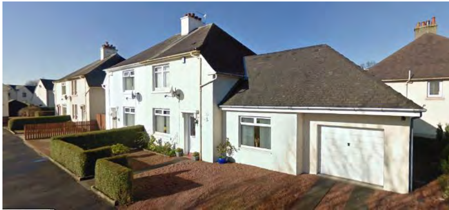
Figure 19: Holehouse Road, Kilmarnock; an example of an extension roof subordinate to the existing one and sympathetic in material and pitch (EAC DP&R).
