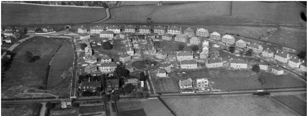
Figure 2: Piersland Park during construction of the second half of the estate (07/10/1927) (Canmore, 2020).
