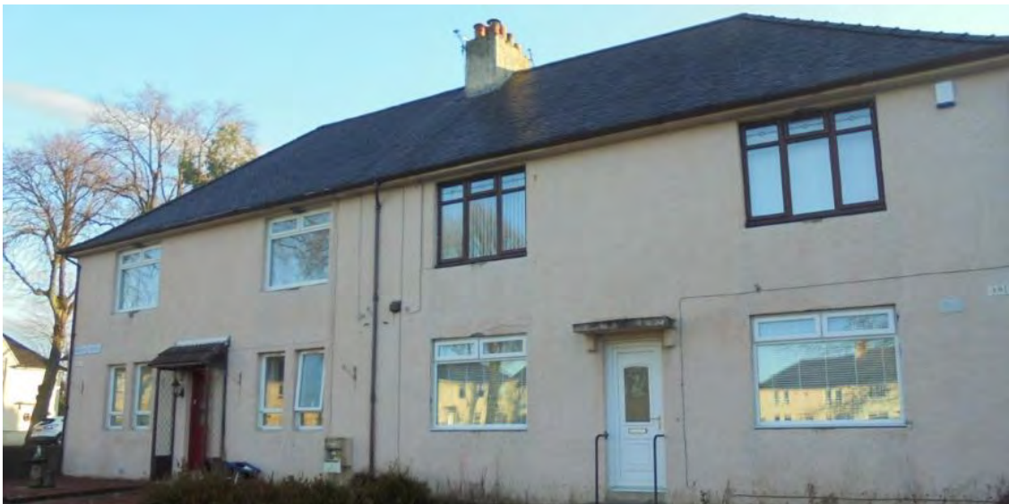
Figure 30: Original windows have often been replaced and mullions were lost, resulting in an incoherent aspect.
