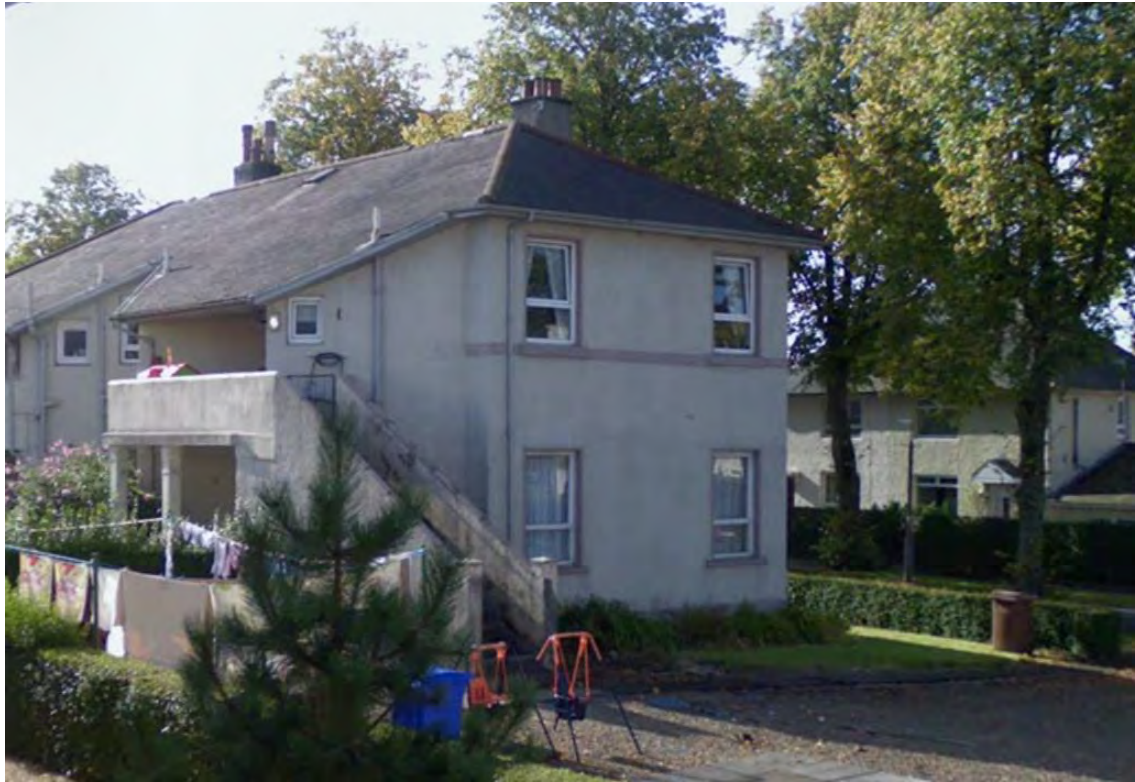
Figure 22: A unique four-in-a-block with deck access.
