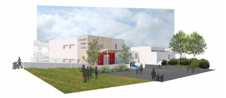
The St Sophia's Primary School project in Galston includes alterations and a deep retrofit which is being delivered to EnerPHit standards. This is a highly sustainable approach applying Passivhaus design principles of super-insulation and air tightness to existing buildings. This approach, which also incorporates a zero direct emission heating system, has the potential to reduce energy demand and carbon emissions by 75% - 90%.
